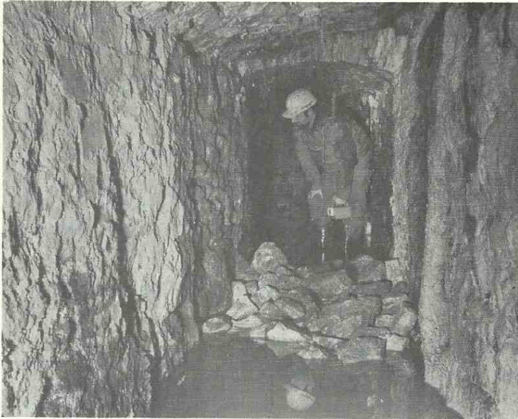
Underground culvert system
